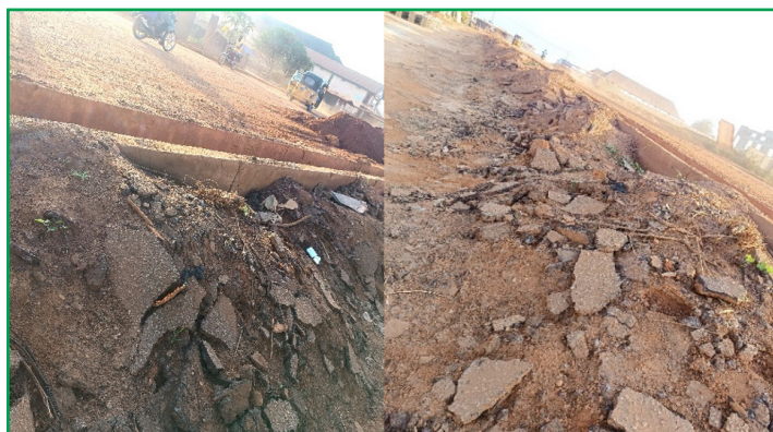
Figure 1. Discarded RAP at Oda Road construction site
