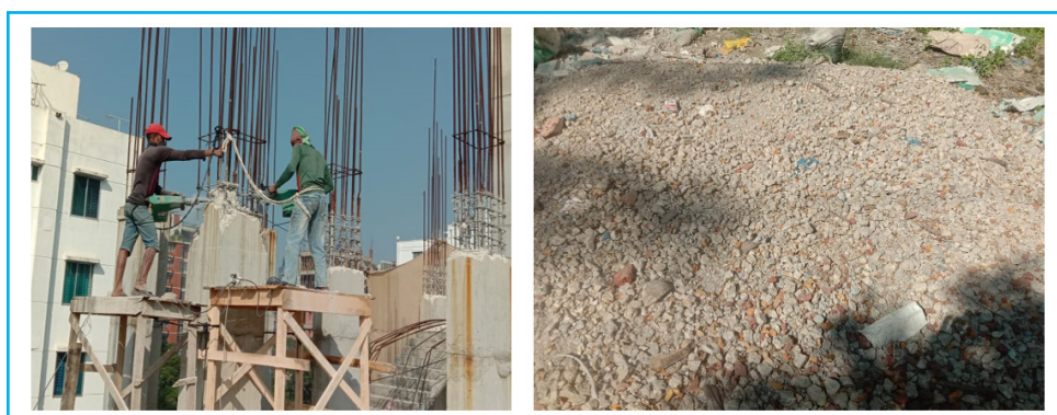
Figure 1. Collaction of column demolished aggregate (Location: Bashundhara RA, Dhaka)
