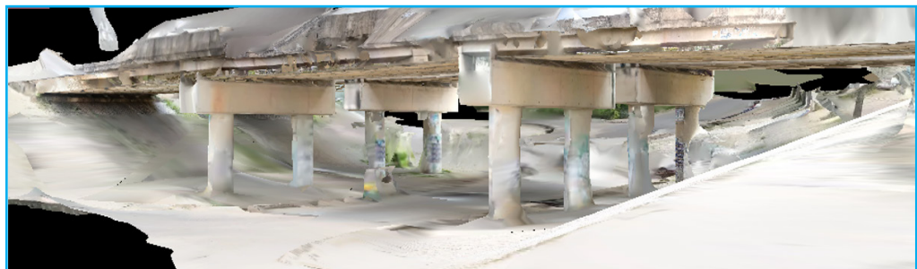
Figure 9. 3D model of the bridge generated by DJI Terra
