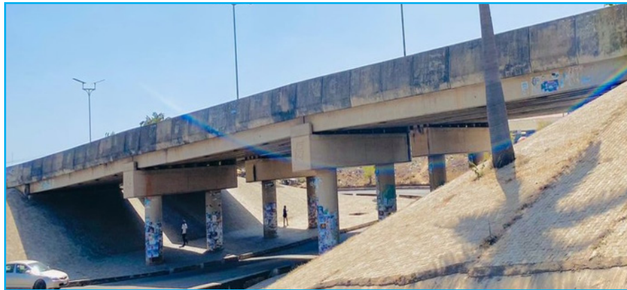
Figure 3. Real image of the bridge
