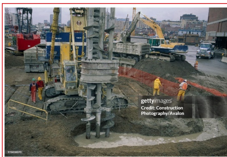
Figure 7. Soil mixing ground support on Boston Big Dig, Central Artery Tunnel Project
