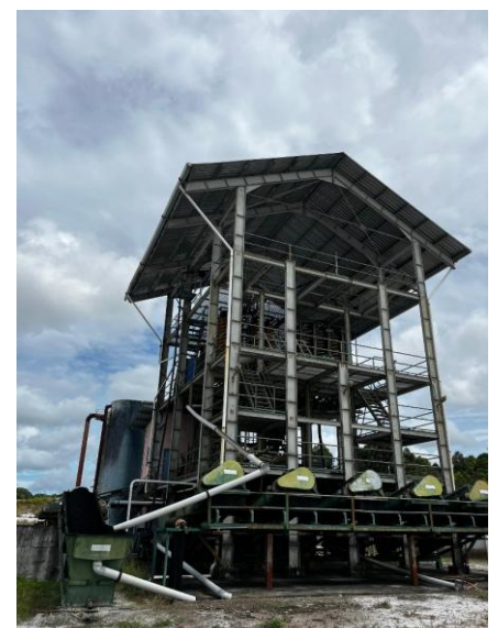
Figure 8. Rear view of inactive silica sand processing plant (MRD01)
